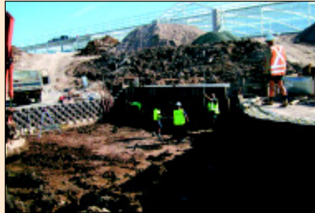
Investigations at Maitland site
