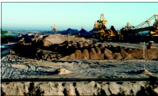
Stage 2 of Preload at the Kooragang Coal Terminal Expansion
