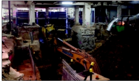
Early stage of car stacker excavation and service passageways
