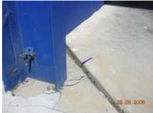
Figure 2: Relative movement between slab and piled column
