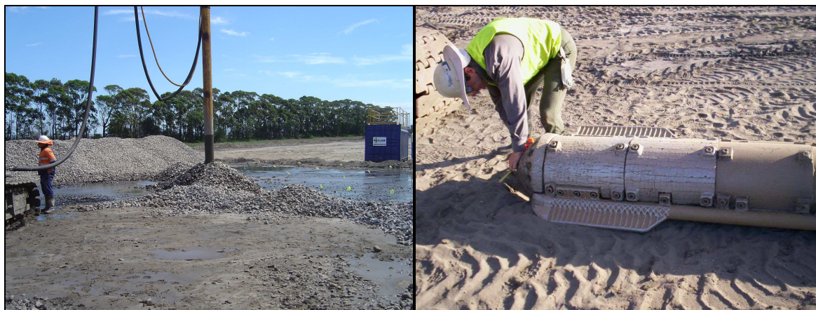
Figure 1: Installation of Stone Columns and Close-up of Vibro-Replacement Probe
