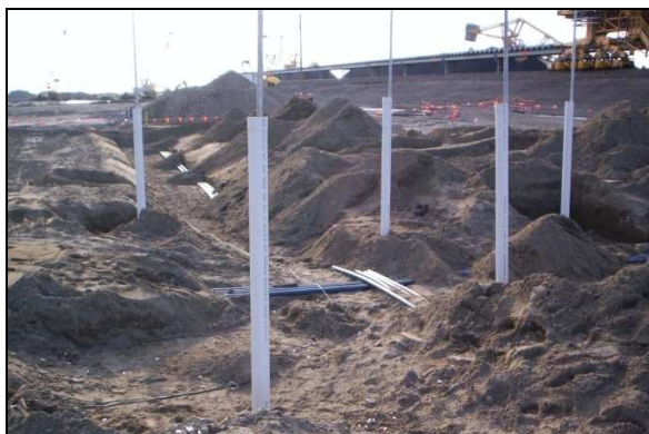
Figure 3: Instruments prior to placing fill
