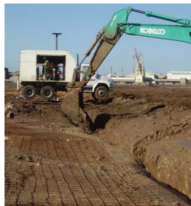
Fig. 8 - CPTu testing on top of barrier wall
