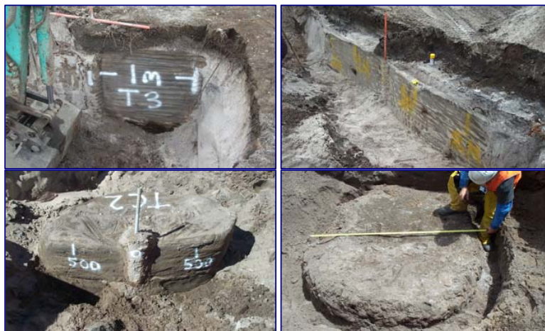
Figure 1: Example of jet grouting shapes (Sydney helipad)
