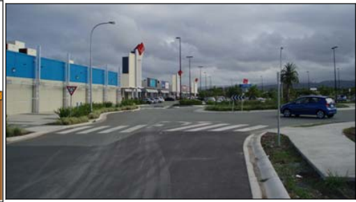
Fig. 7 View of the project at transition area three years after construction
