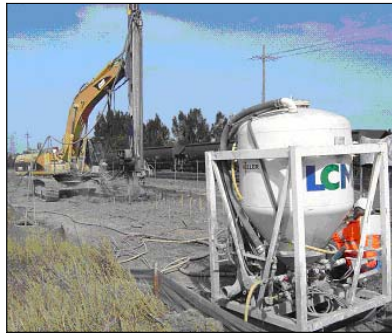
Fig. 3 - View of the site installation
